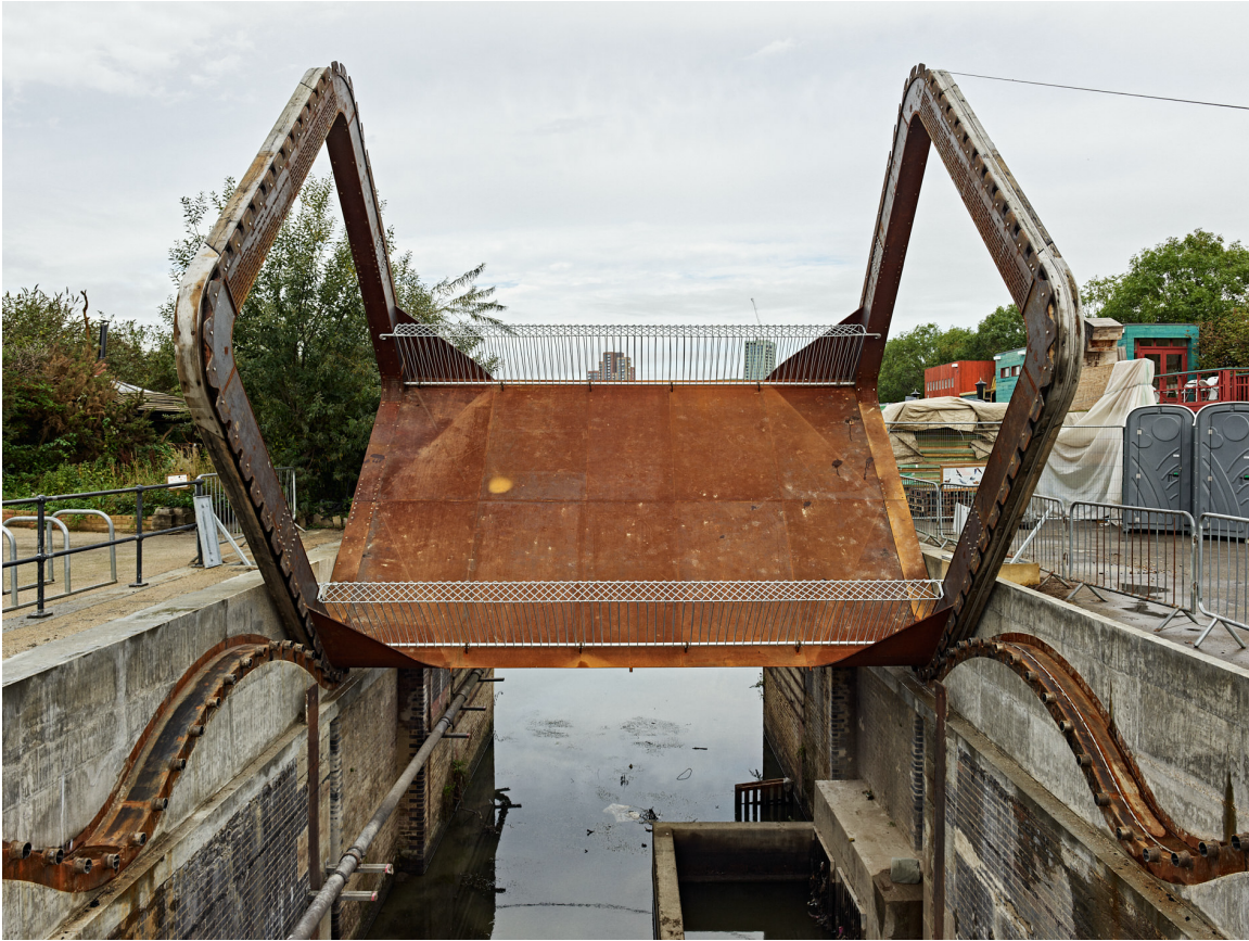
Figure 7. The Cody Dock bridge rolling along catenaries toward its upside-down position along. Photo by G. G. Archard.
